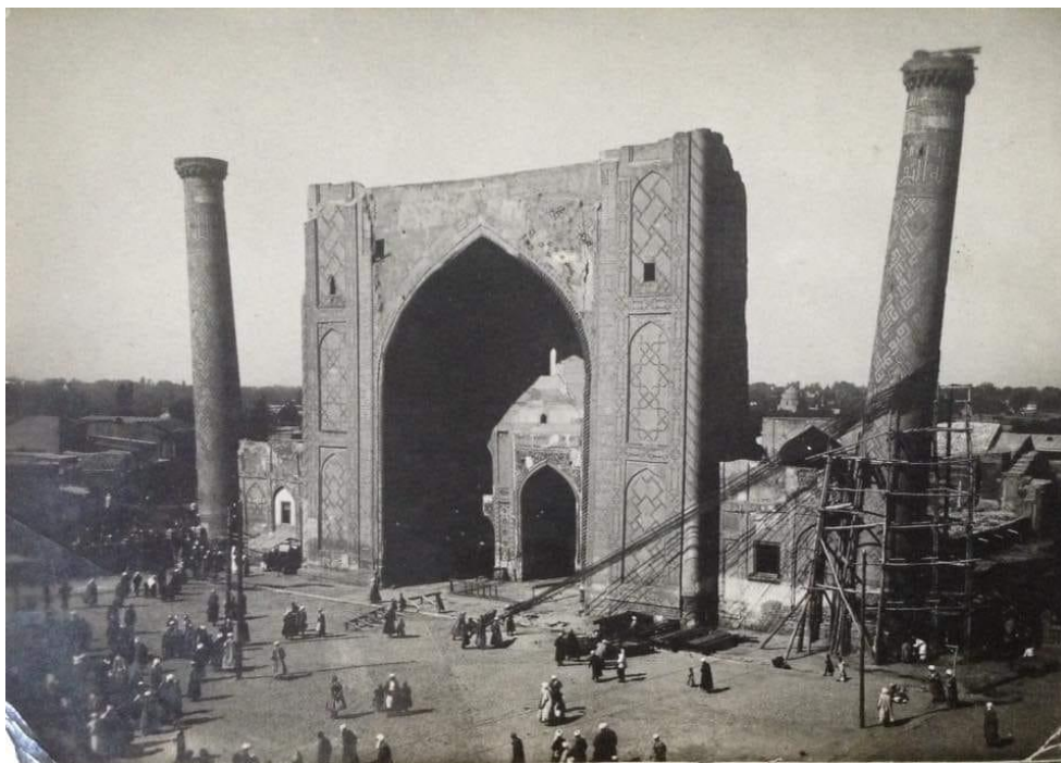
Figure 1. The minaret, weighing 36 tons, was reinforced with 24 iron cables, stretched from its base
