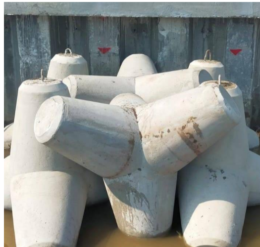
Figure 2. Tetrapod Arrangement (interlocking)
