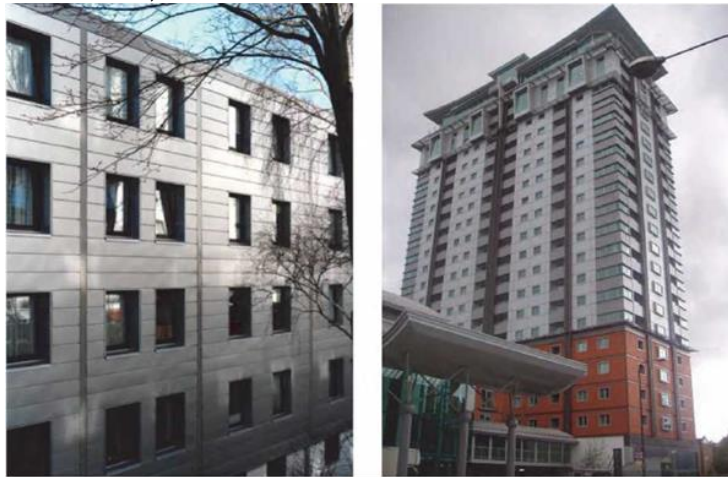
Figure 1. Examples of installing new facade systems on old facades of buildings with concrete wall panels. The new facade systems consist of horizontal metal panels
