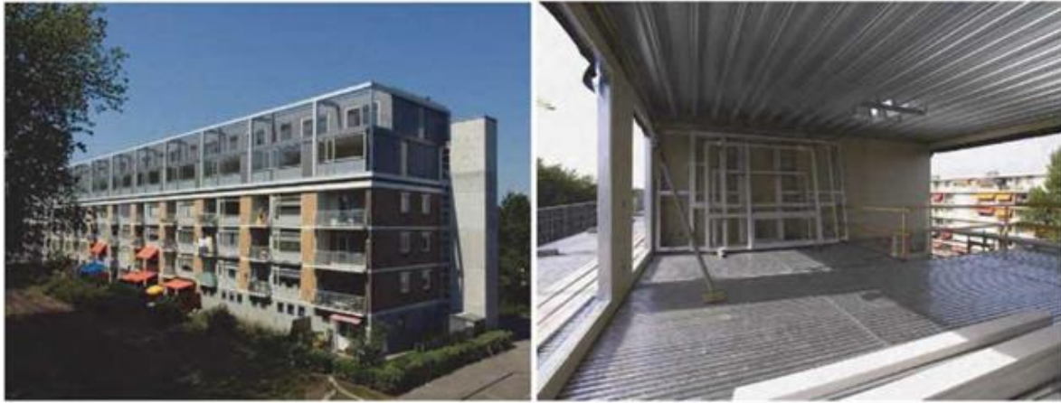
Figure 2. Two-storey superstructure made of light steel frame on an existing building, Rotterdam
